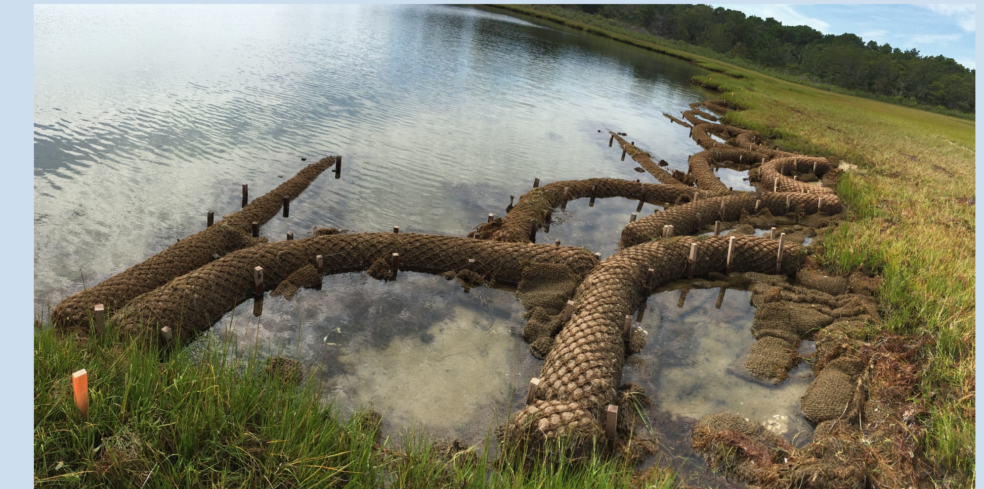
Living shoreline installation on Sengkontacket Pond
